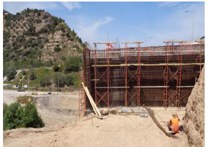
B269 – Construction of left backwall
