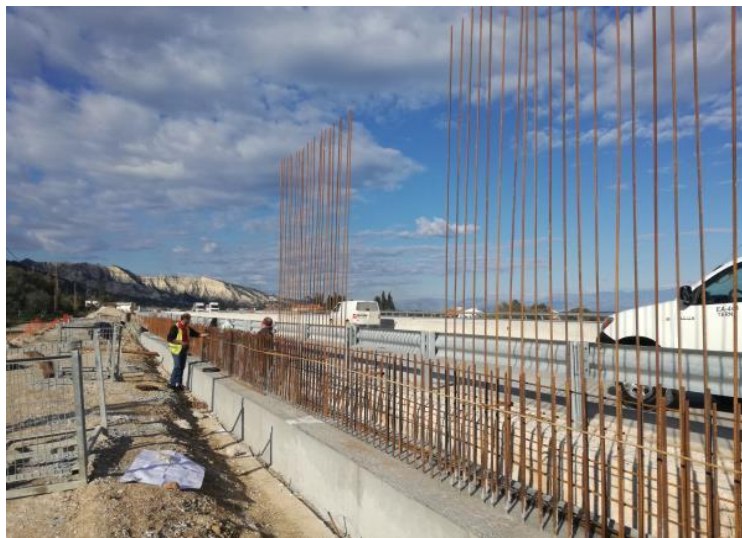
Construction of noise barriers at k.p. 39+776.5 to k.p. 39+835
