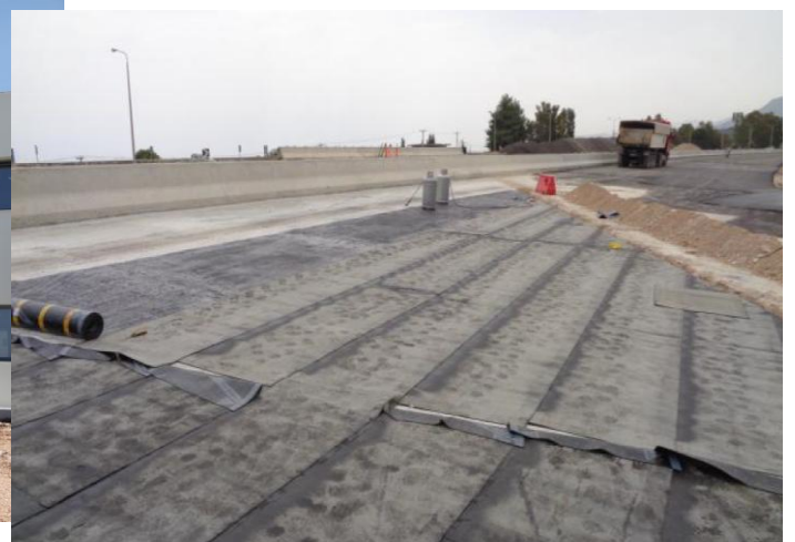
K317 – Installation of deck slab waterproofing
