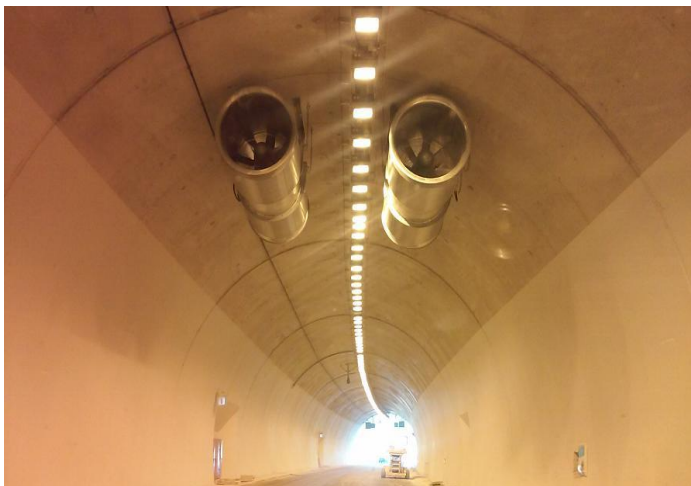
Tunnel Akrata 13A – Ventilation system
