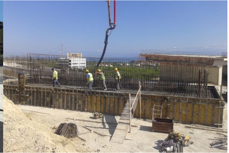
Overpass A215 – Pouring abutment A2
