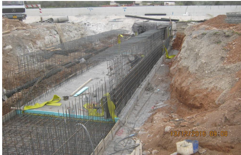
L218 – Construction of box culvert
