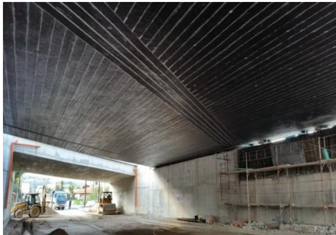
Completion of FRP strips installation at K305
