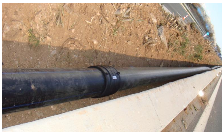
Installation of irrigation pipes
